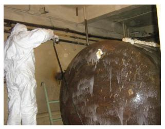
Figure 5. Applying polymer localizing coating.
