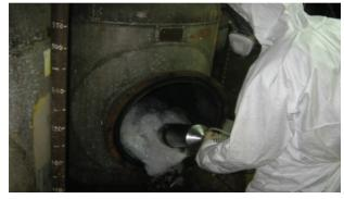
Figure 8. Foam decontamination of the internal equipment surfaces.
