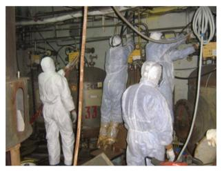
Figure 2. Dismantling the process pipelines.
