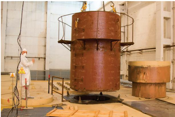
**Figure 4.** K-1 cask positioned above the storage compartment.
