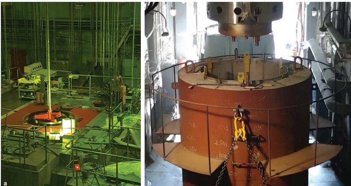
**Figure 2.** SM-3 reactor core withdrawal. **a.** From the reactor cavity; **b.** Loading into the K-1 cask.
